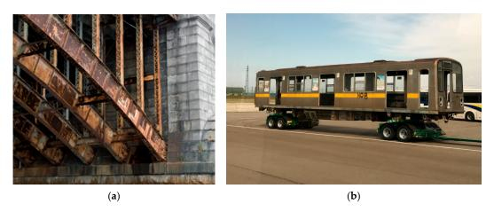
Figure 8. Corrosion of steel. (a) Extreme corrosion in a bridge. (b) Railway rolling stock being renovated.
