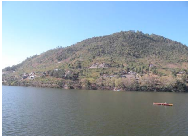
Image 3. Looking west over Bhimtal Lake, showing ongoing urbanization on Jones Estate watershed in January 2012.
